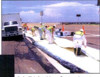
Poly-Triplex Liner System is saturated with epoxy resins and prepared to be inserted into the deteriorated culvert.
