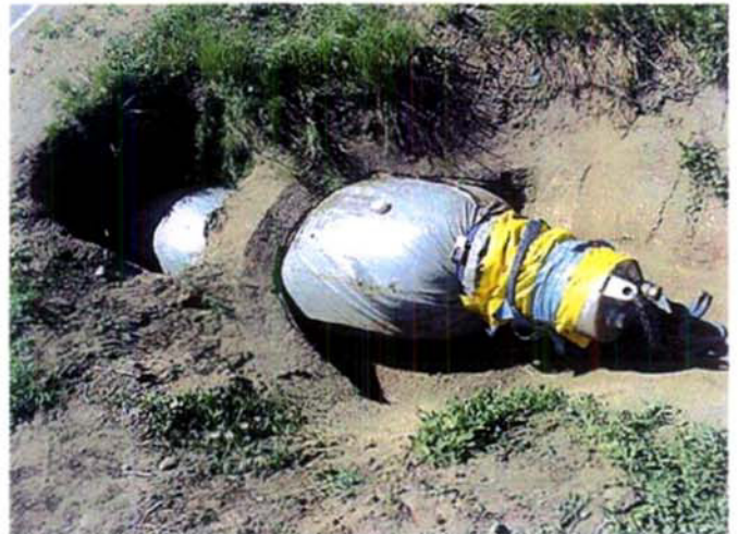
Poly-Triplex® Liner Curing (approx. 3 hours).
