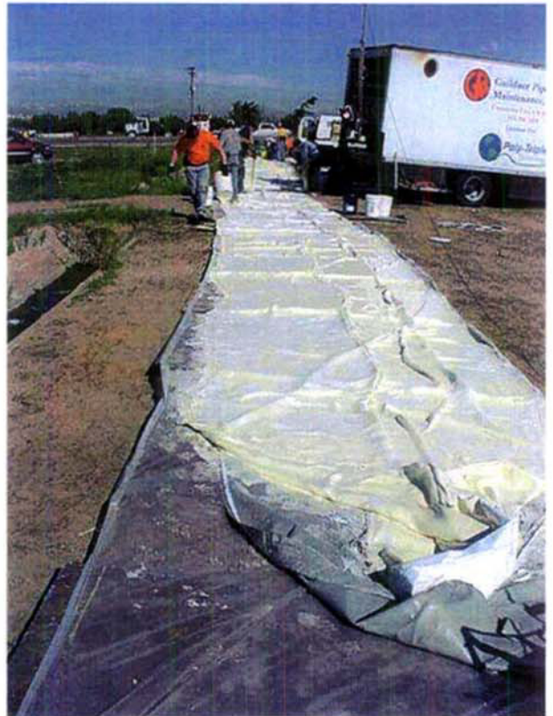
Epoxy Resin applied to Liner prior to installation.
